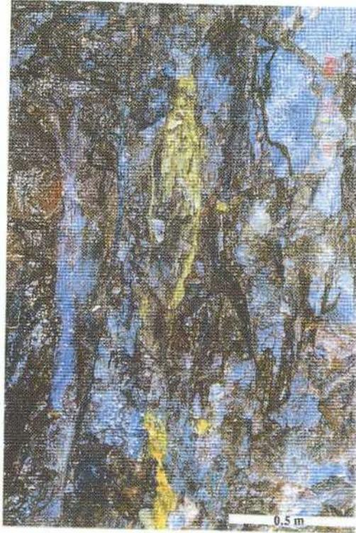
**Figure 2-10a.** Fracture zone NNW-4W. Intersection the tunnel at 2018 m. The yellow fracture filling is coloured grouting material /Photo K Annertz/.
