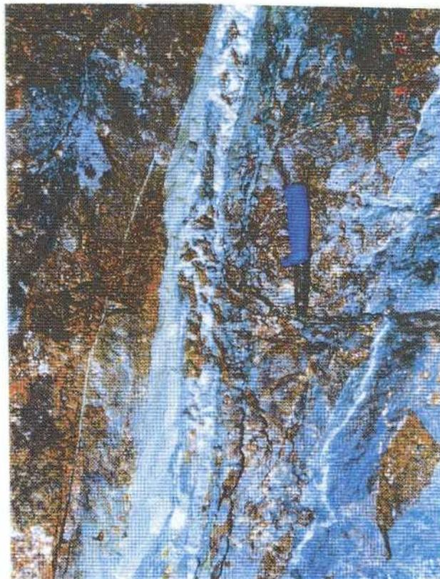
**Figure 2-10b.** Fracture zone NNW-4W. Intersection the tunnel at 2116 m. White fracture filling is calcite, grey is grouting material /Photo K Annertz/.
